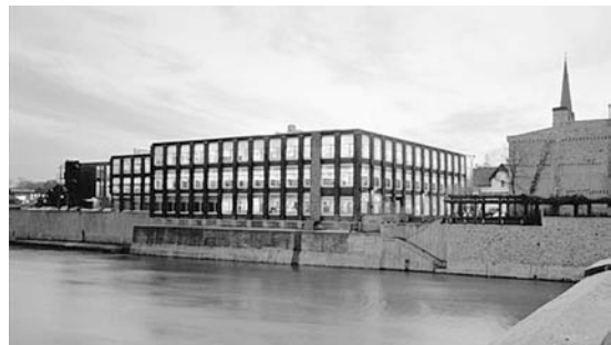
FIGURE 10. The University of Waterloo School of Architecture building in Cambridge, Ontario, was insulated in part with rigid foam board insulation on the interior.
